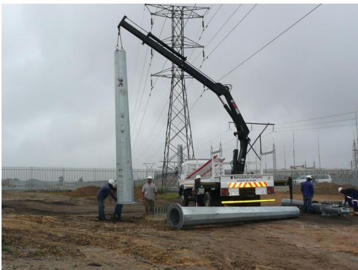
Picture: 66 kV Mono Pole Installed:
