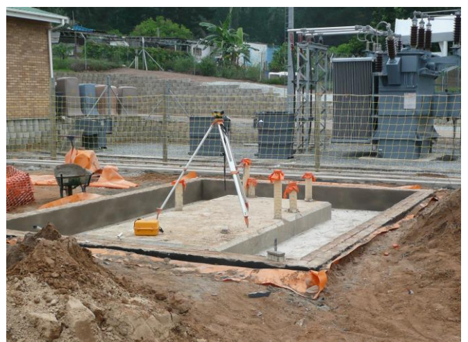
Picture: Trf plinth under construction
