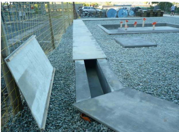
Picture: Trf bund wall and oil sump
