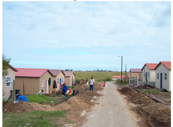
Picture: Trenching for feeder cables
