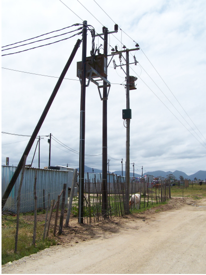
Picture: Pole top box for service connections
